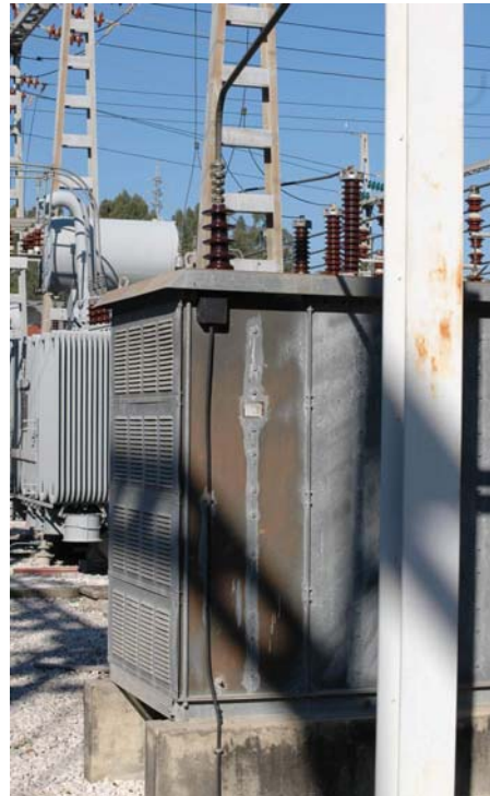
Figure 8: Neutral Resistor box
